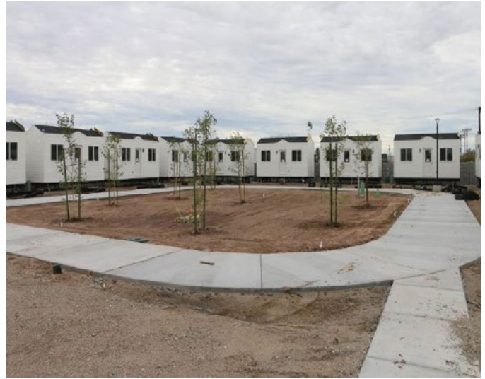
Tiny homes under construction at Imperial Valley College's Lotus Living community.
